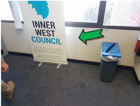
Photo 7. Interior, throughout, beneath windows, walls – non asbestos-containing fibre cement sheeting.
