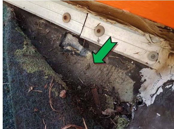
Photo 2. Exterior, level 1, terrace, waterproof membrane – non asbestos-containing bituminous material.
