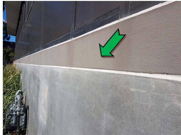
Photo 4. Exterior, throughout, walls – non asbestos-containing mastic sealant.
