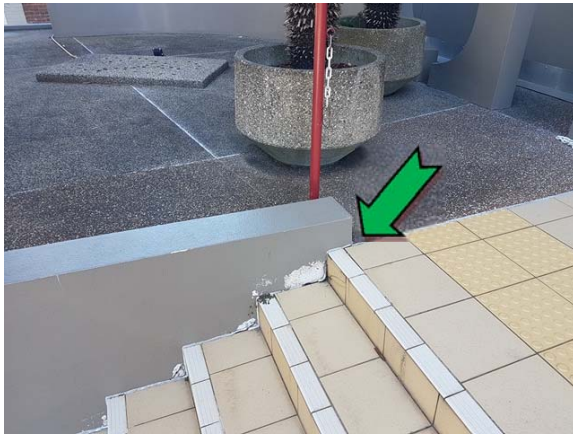
Photo 3. Exterior, throughout, entrance stairs, expansion joint – non asbestos-containing mastic sealant.
