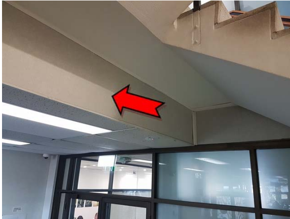
Photo 13. Interior, level 1, ceiling space, infill panels – suspected asbestos-containing fibre cement sheeting.
